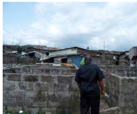
Typical 3 sqm room block with central access under construction
